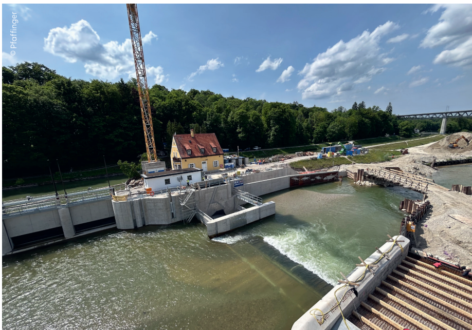
The construction site revealed some surprises.
