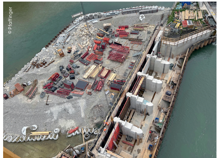
Bird's-eye view of the weir piers at the new diversion weir
