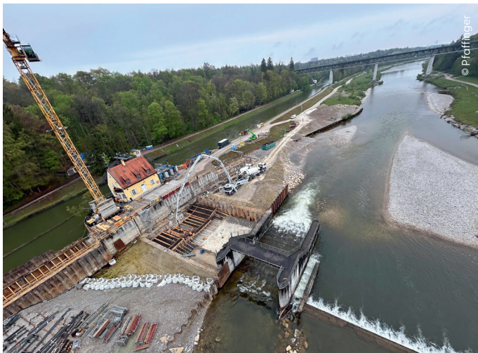
Concreting work on weir section 1
